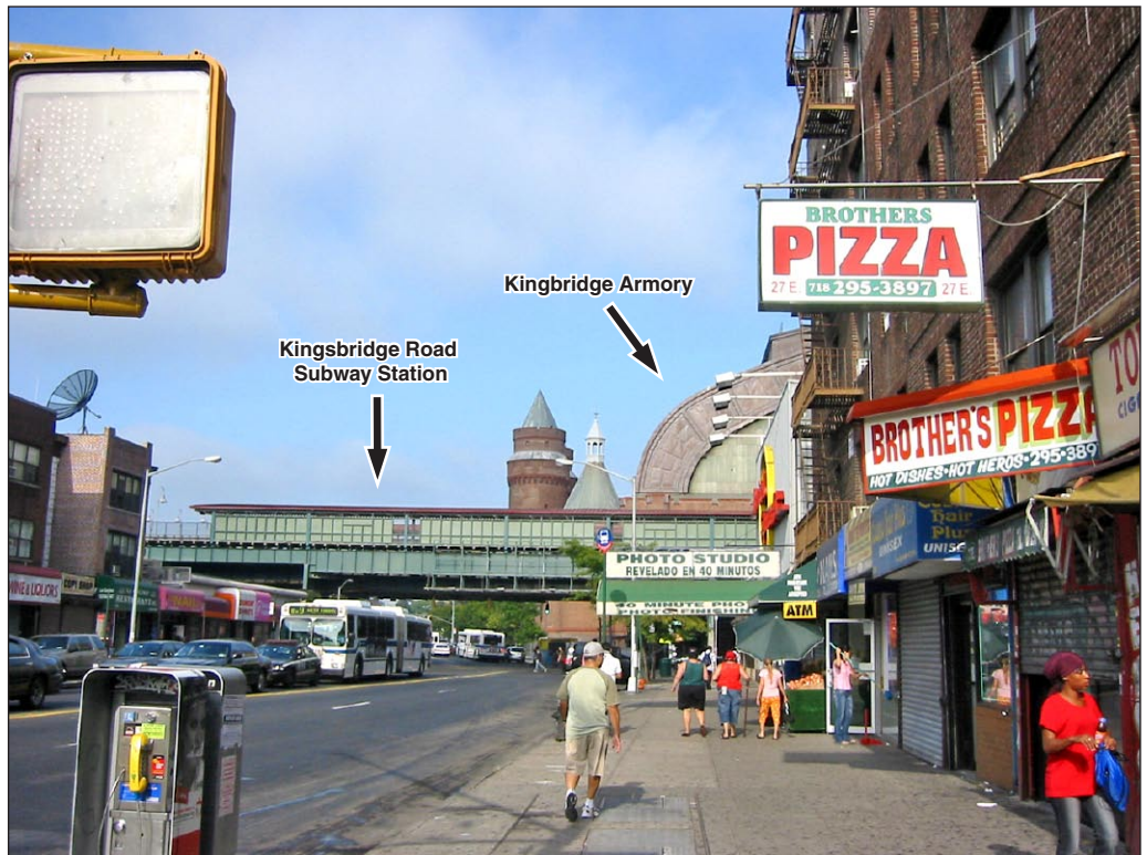
View west on East Kingsbridge Road to the Kingsbridge Road subway station
