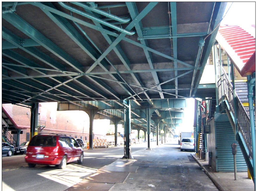
View north on Jerome Avenue - Kingsbridge Road subway station viaduct and platform above
